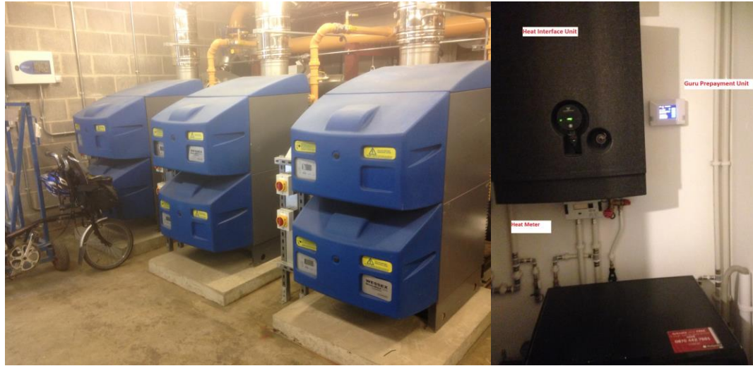
Communal boiler plus HIU 28% to 75% efficient
